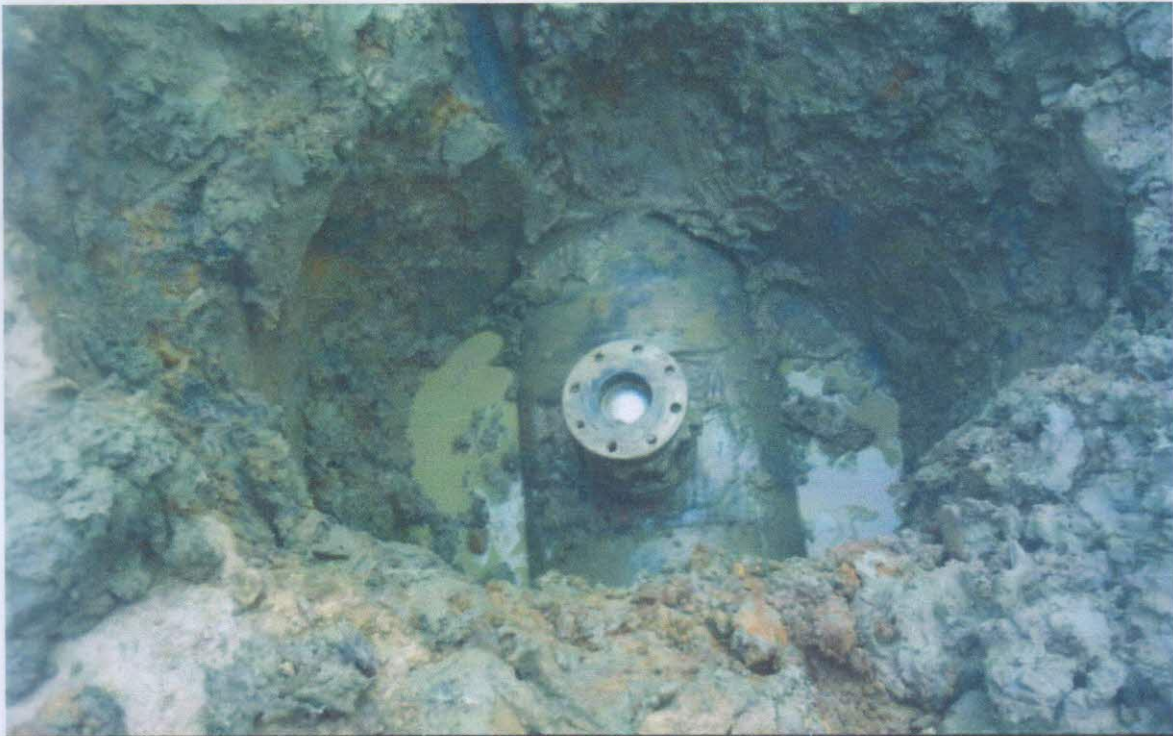
PIC ONE: BEFORE EXCAVATION
